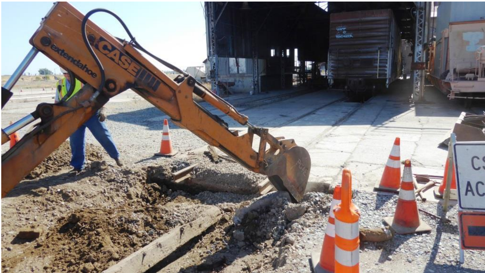
Harry uses the extendahoe to break away a large chunk of concrete from the end of the rail
