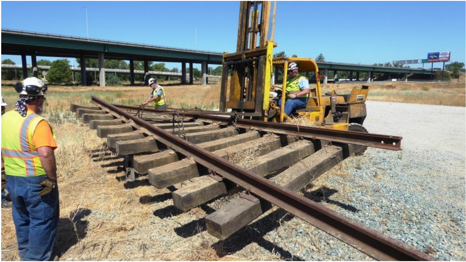
Chris, on the 15,000-pound forklift, moves the track panel to the prepared roadbed
