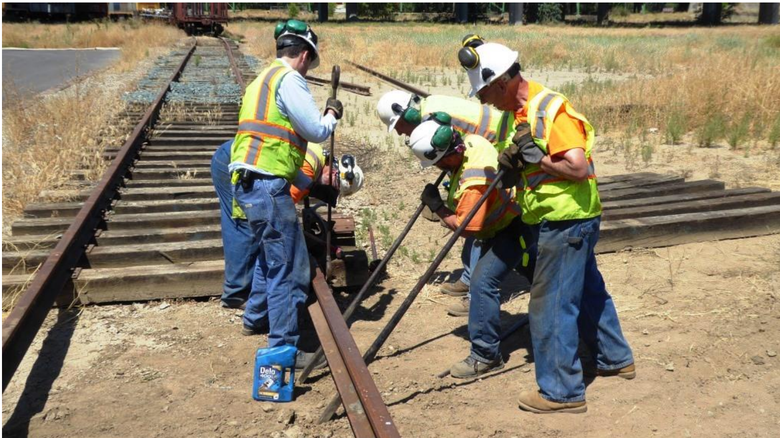
Weston tightens the bolts as Joe and Clem hold the rail in place with lining-bars
