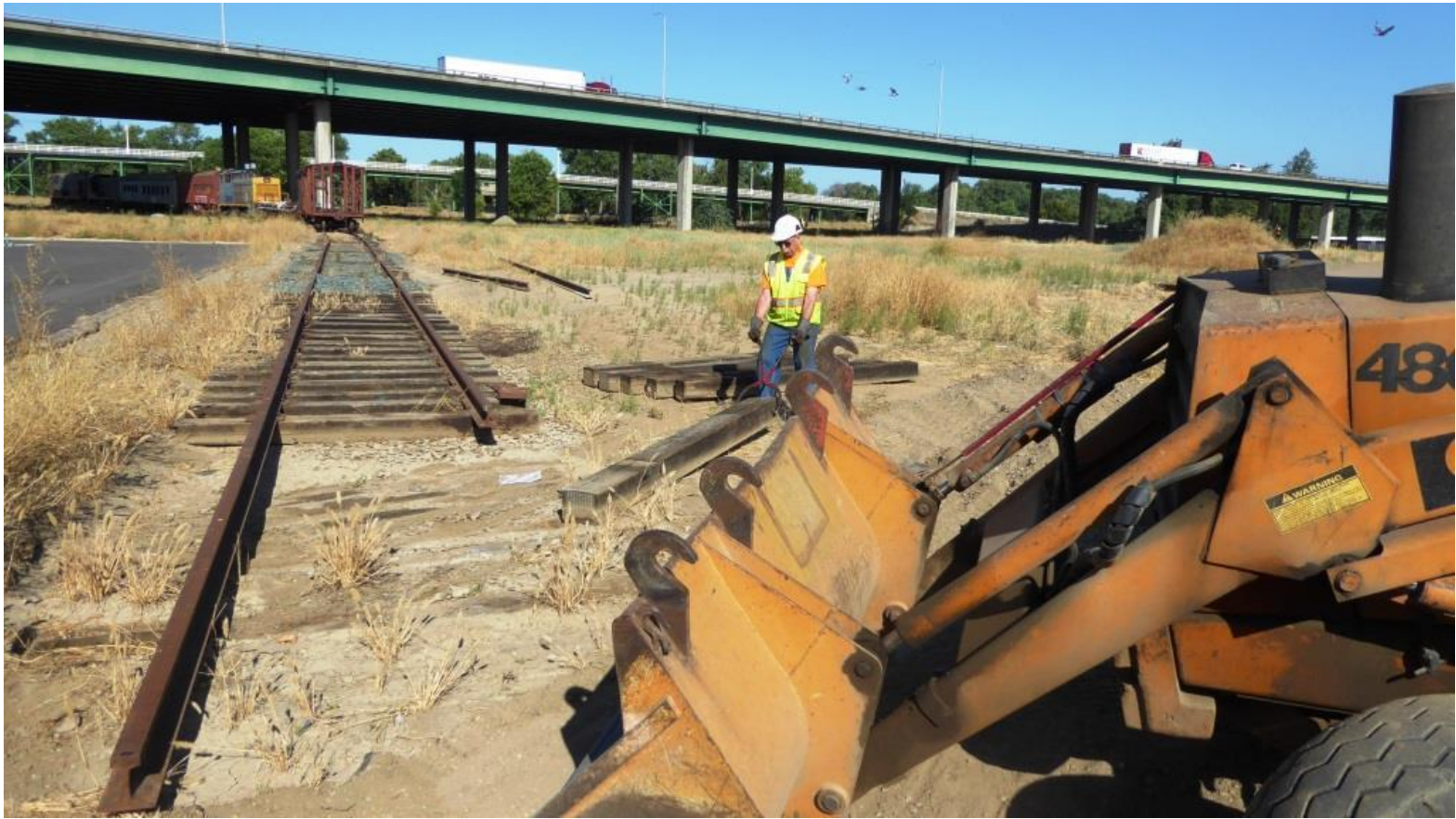
Thanks to Clem, the ties were out of the way for Harry on the back-hoe to come in and lower the roadbed
