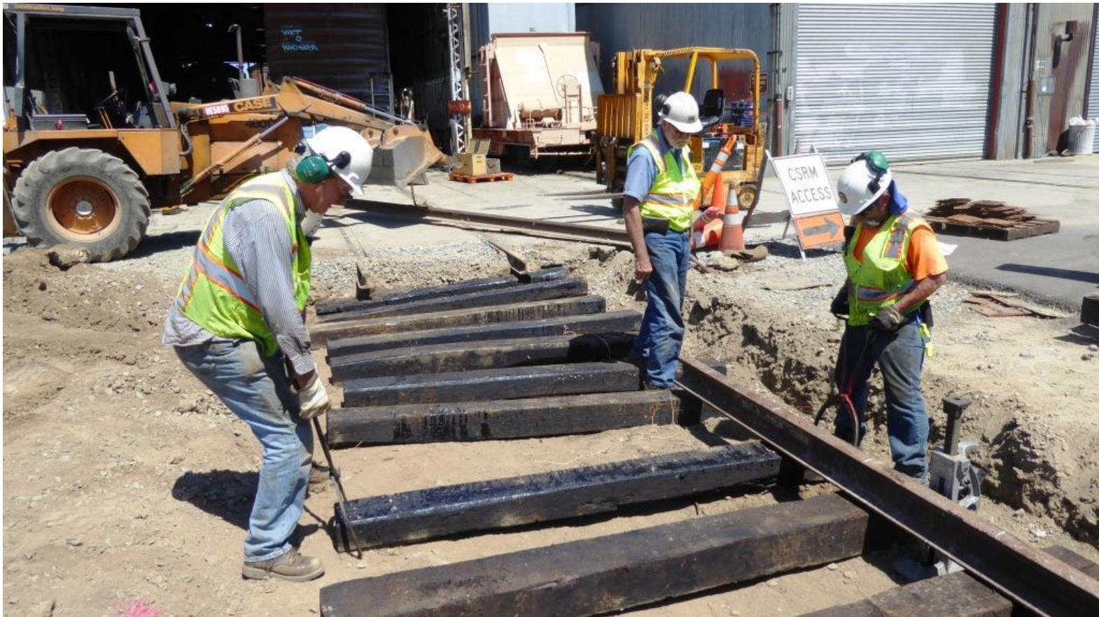
Steve and Joe arrange ties under the rail
