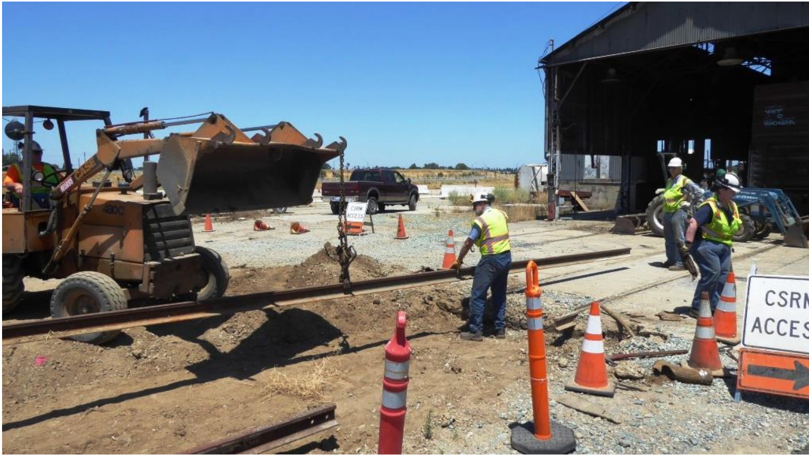
Harry on the back-hoe brings in the next stick of rail which needs to be cut
