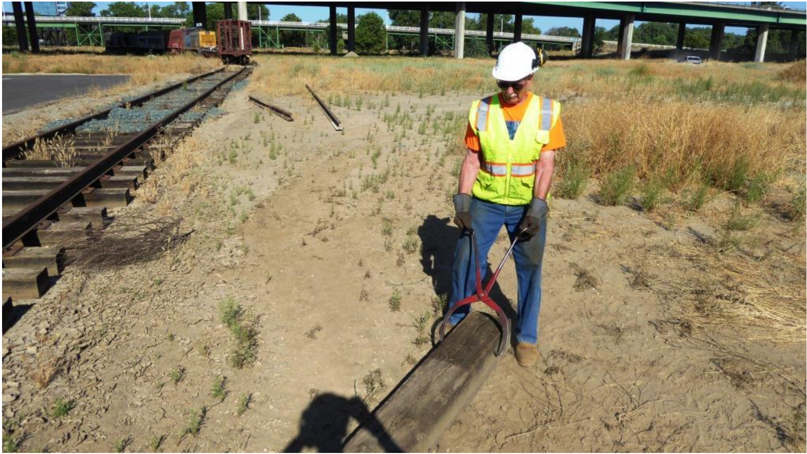
Clem moves a heavy oak tie out of the way
