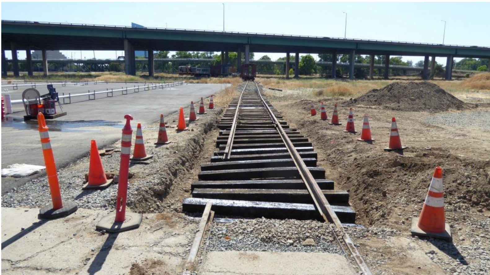
Well, it's starting to look like a real track – a little leveling, surfacing, ballasting, spiking, and tamping is all it needs...
