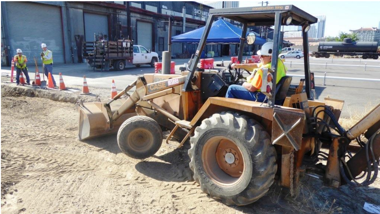
Wheelies with the back-hoe! Harry uses the bucket as a grader to level the roadbed
