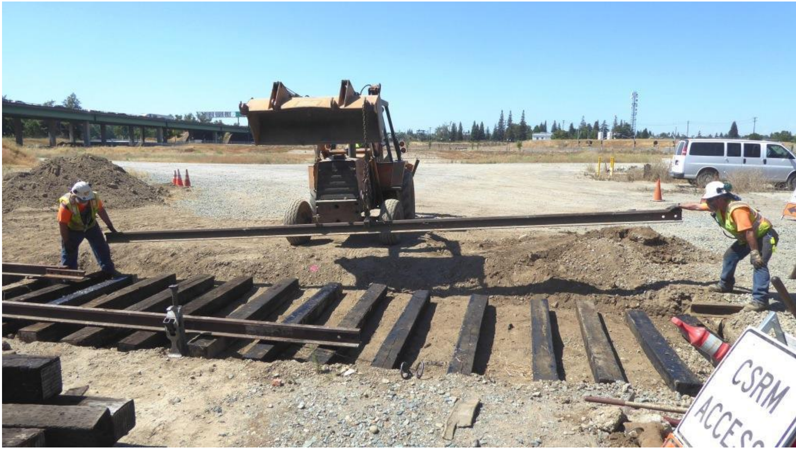
Mike and Joe position the freshly cut gap-rail into position
