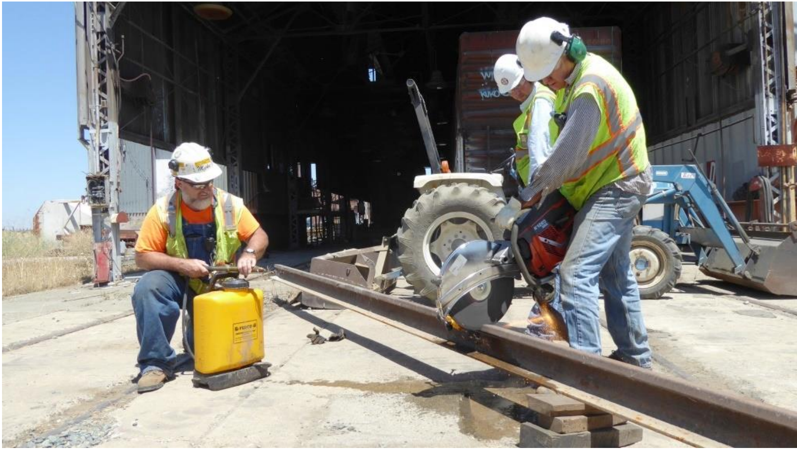
Mike at the ready with the Indian Pump as Steve cuts and Weston handles the spark-shield
