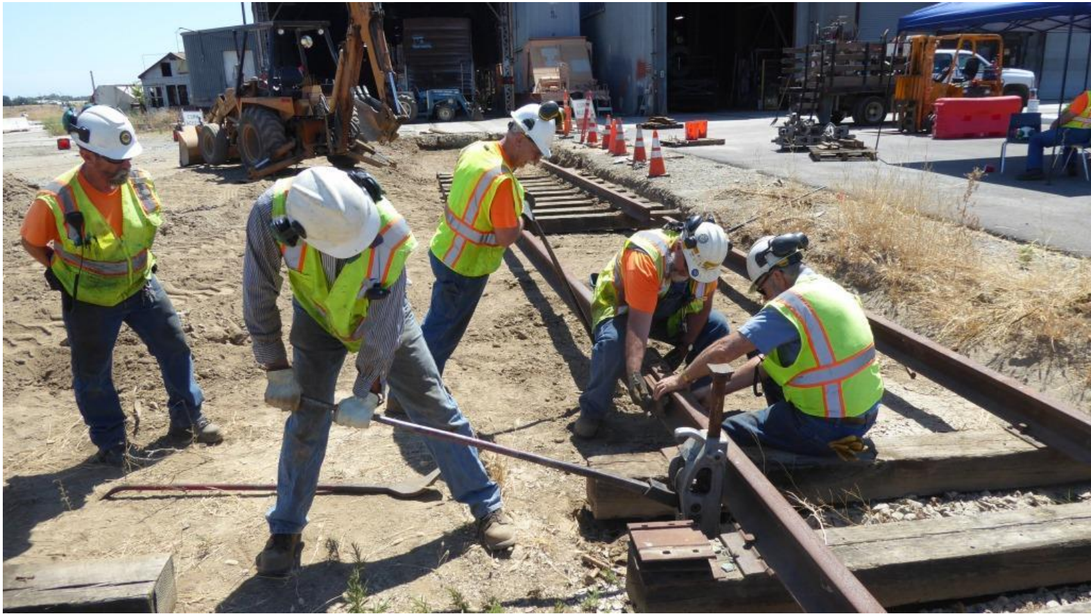
Steve raises the track vertically with a jack as Clem pushes it horizontally to line up the rail-ends for Alan and Mike to bolt in a joint bar
