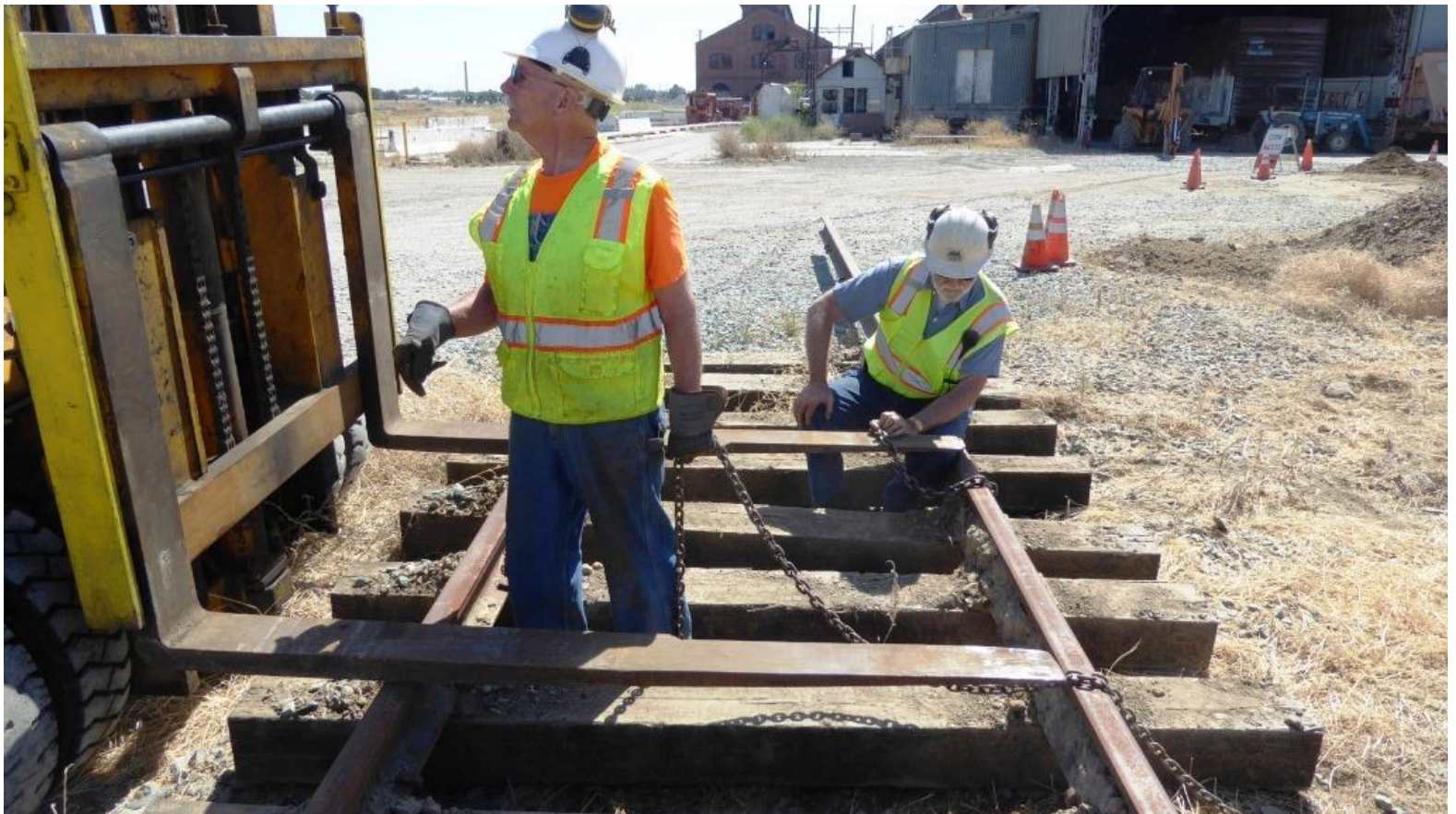
Clem and Alan chain the panel to the forklift
