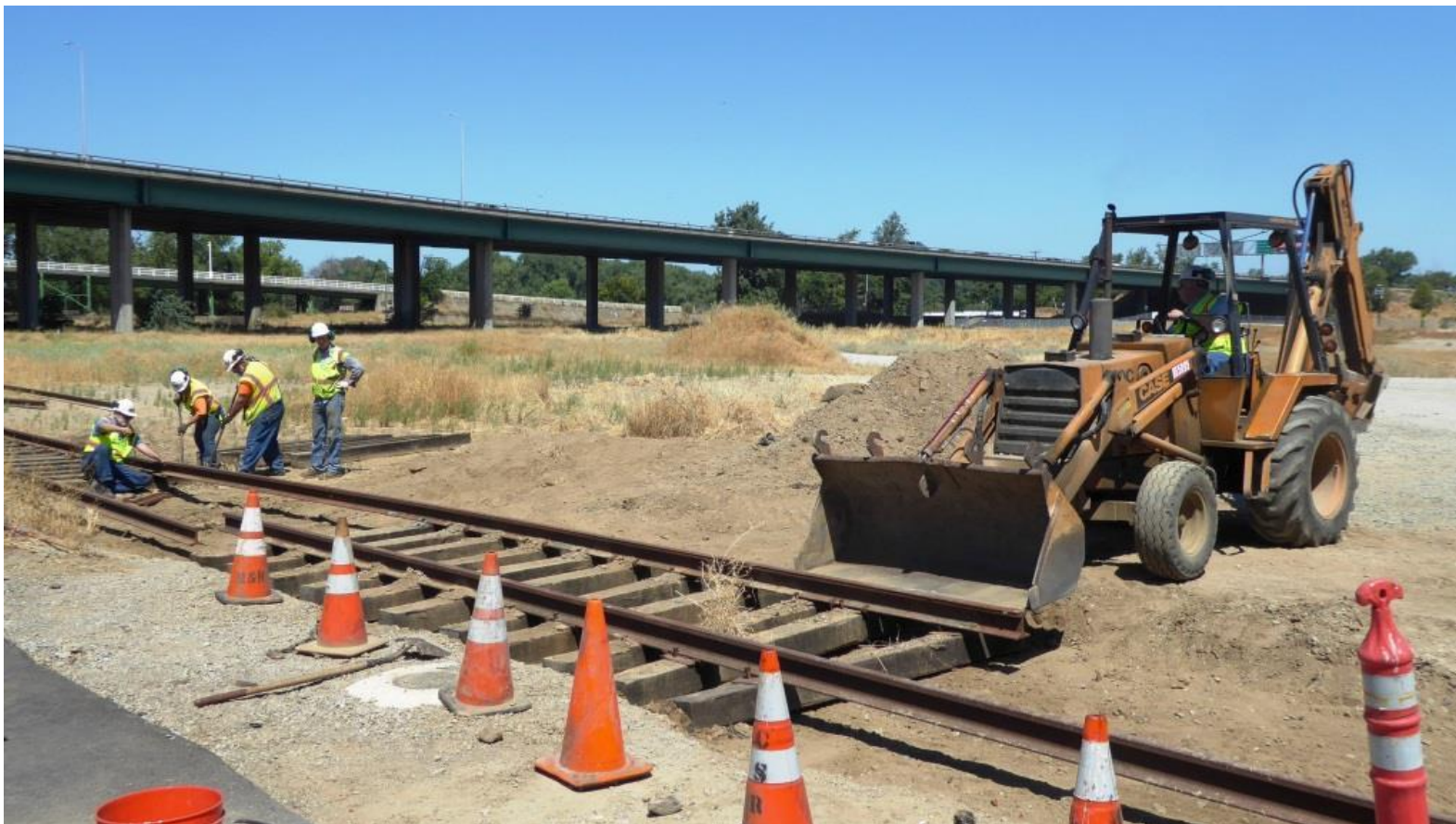
With a little help from the back-hoe, the track is shimmied about a bit to get the rail-ends to match up
