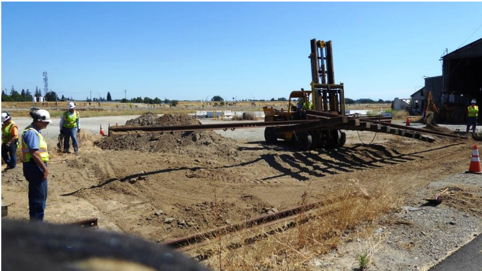
The track-panel is ready for placement
