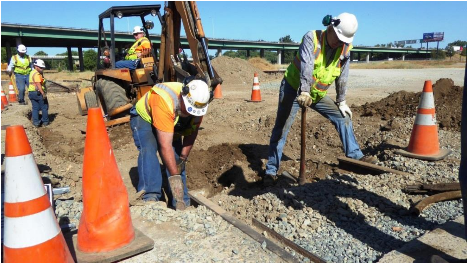
Mike and Steve remove dirt and debris from the end of the Firing Line track where the connection with the storage track will be made
