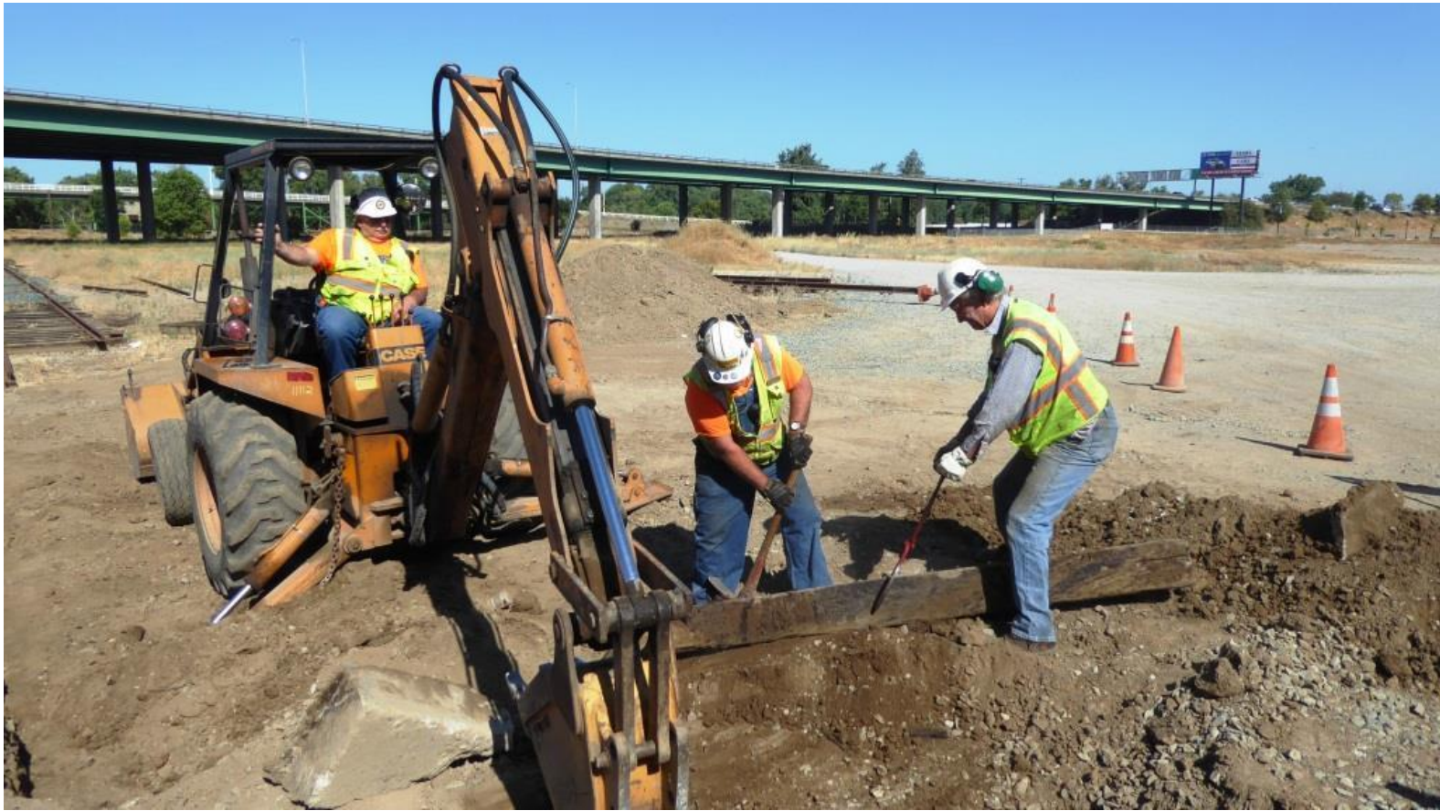
Mike and Steve remove a rotten tie that had been half-buried in concrete for 50 years
